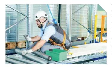
The same applies for repair work, f. ex. on damaged conveyor rollers or brake rollers. After all pallets have been removed from the "trouble" lane, a properly secured assembly person can safely access that lane via a maintenance platform and walk in on the access boards.
