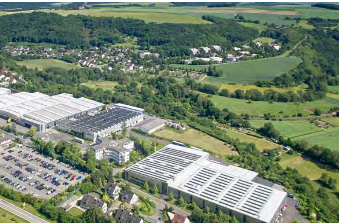
BITO Meisenheim – Headquarters and plant for steel shelving & racking
