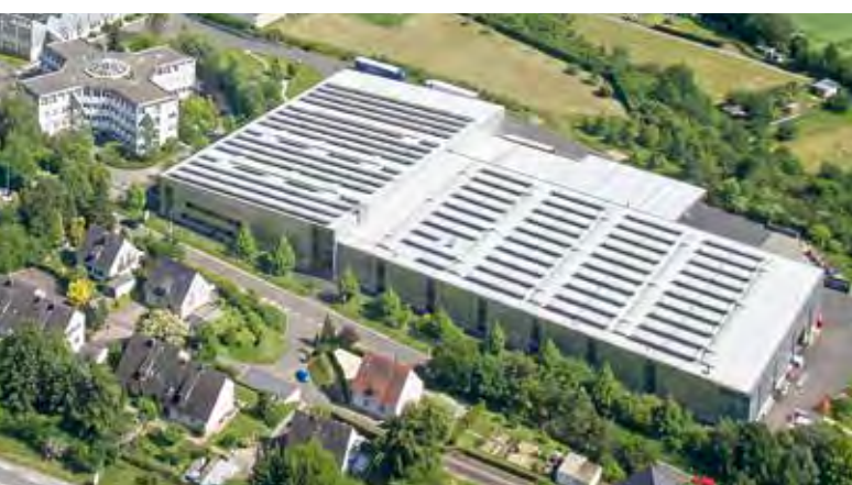
BITO Meisenheim - Photovoltaic panels on plant roof
