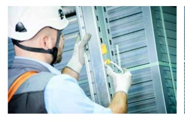
1. Select a safe anchor point for fitting the BITO easyHOOK, lock in the twistlock carabiner.
