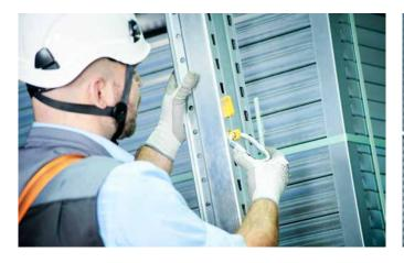
1. Select a safe anchor point for fitting the BITO easyHOOK, lock in the twistlock carabiner.
