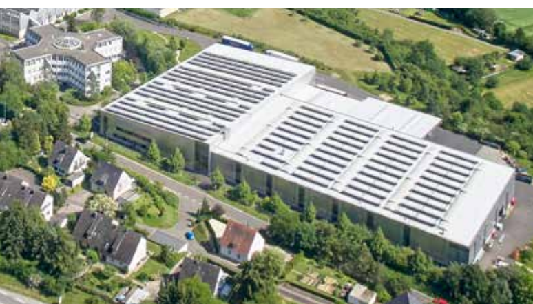
BITO Meisenheim – Installation photovoltaïque
