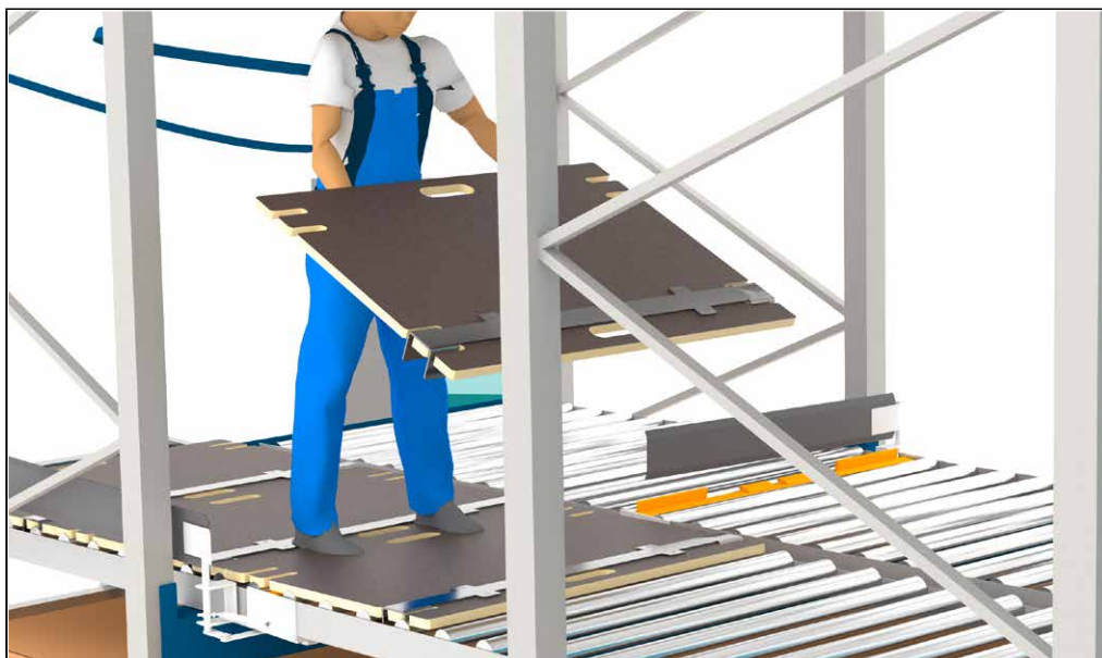
Figure 27: Placing connecting boards
