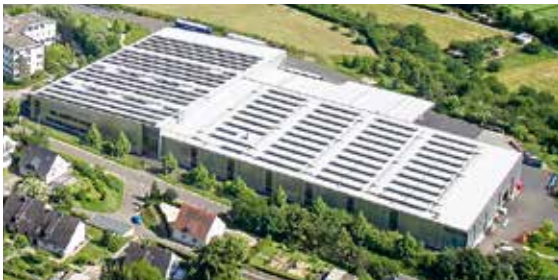
BITO Meisenheim - Photovoltaic panels on plant roof
